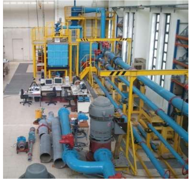
Figure 26: Hydraulic Metrology Laboratory (view).
